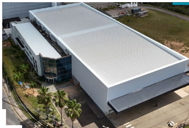
Our new facility and expansion project, Vinhedo II, Brazil.
